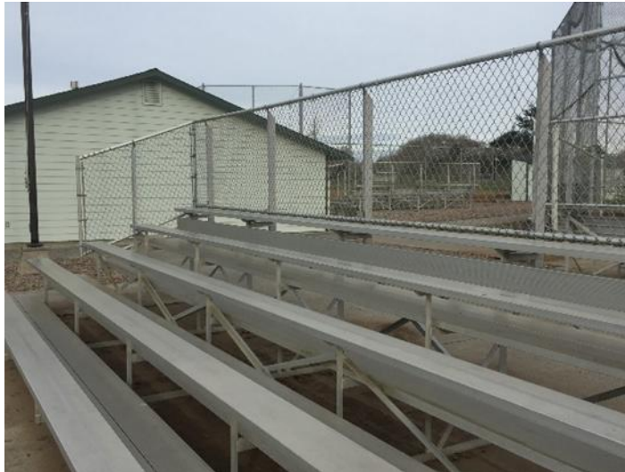
Guard rails provide spectator safety in the bleachers.
