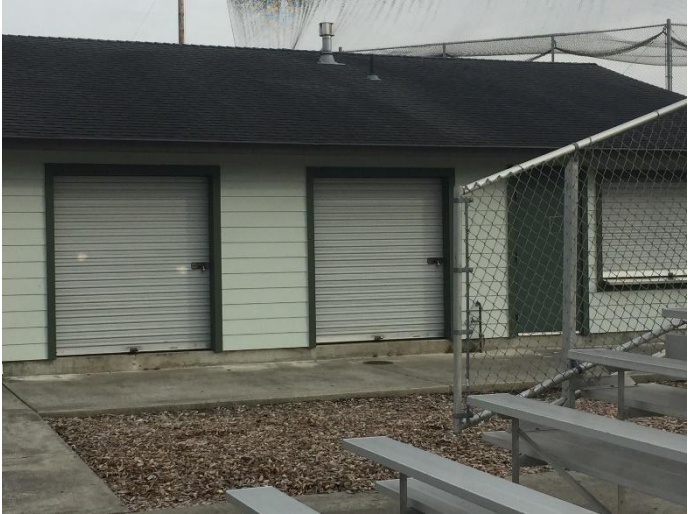
Concession facility and equipment rooms must be locked when not in use.
