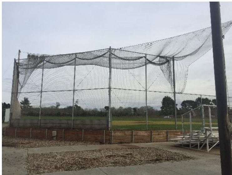
A large backstop with protective screening prevents spectator injuries from foul balls.
